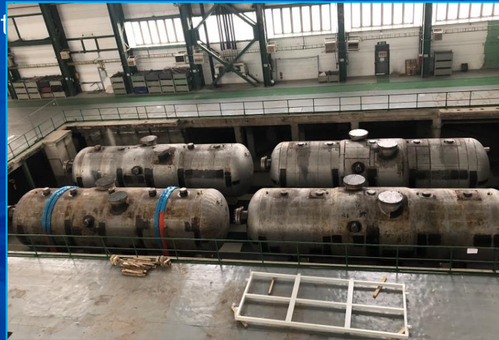
Established SG storage area
