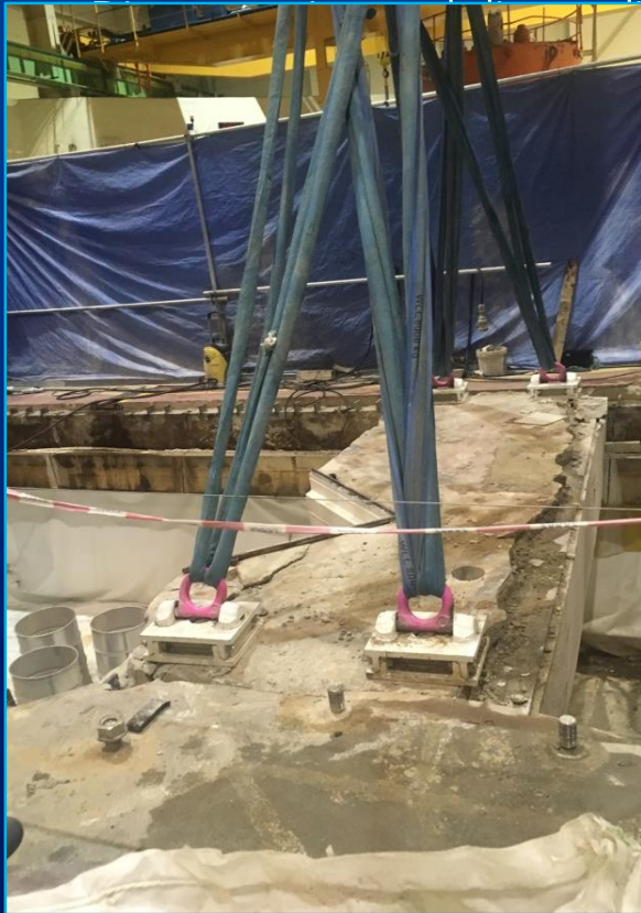
Removal of slab
