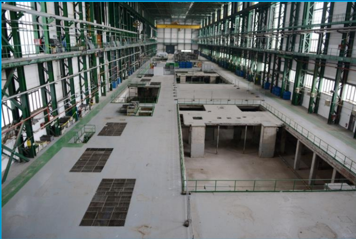
Demolition and establishment of storage and est
